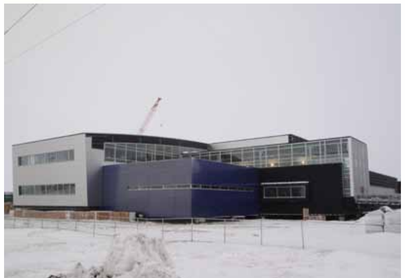
Construction of the new hospital, Winter 2011
